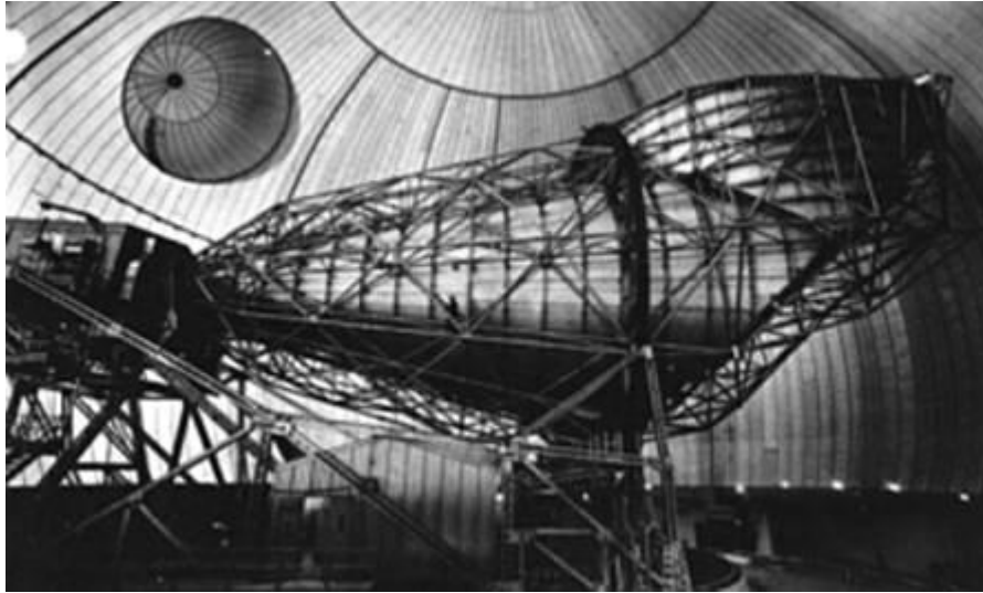
Figure 11. Antenna at Andover, Maine, USA, 1961.
